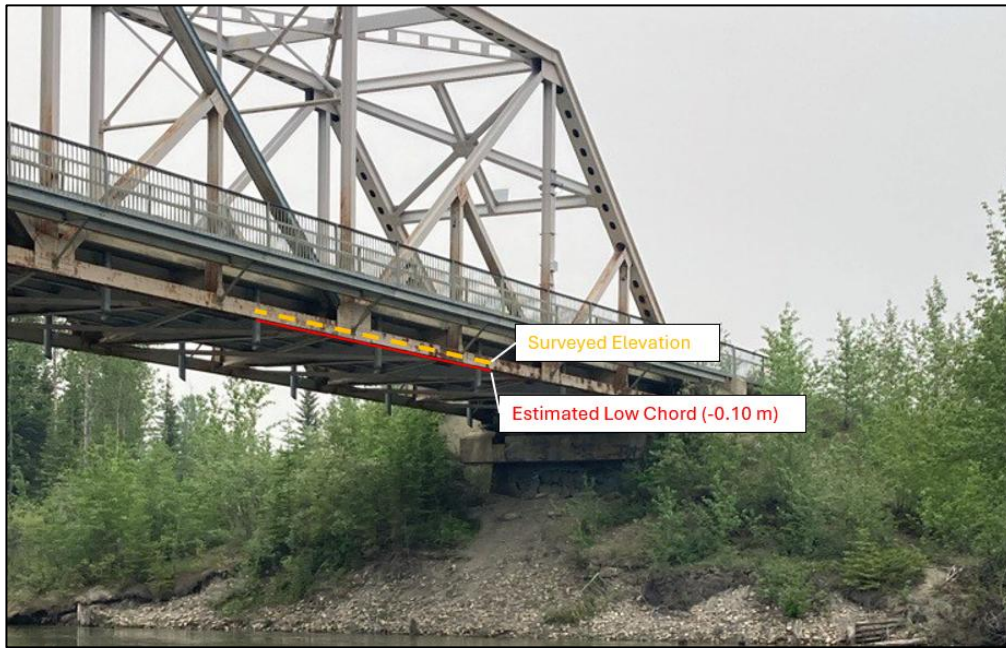
Figure 7-3 – Estimated Bridge Low Chord
