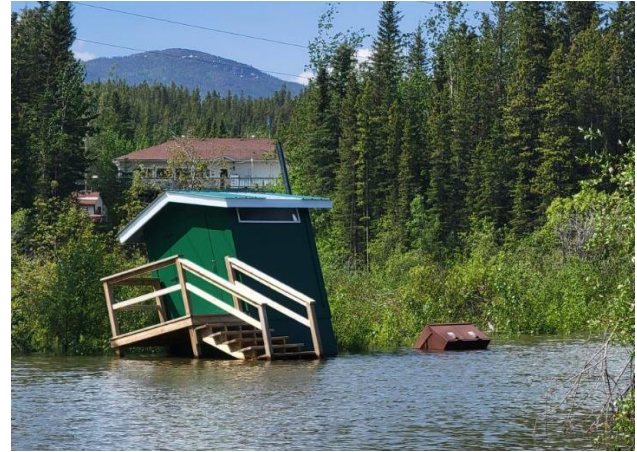
Johnson's Crossing boat launch (2022 Flood)
