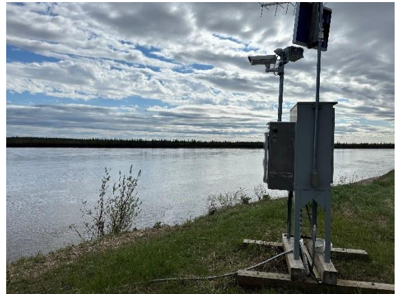
Water Survey of Canada station in Old Crow
