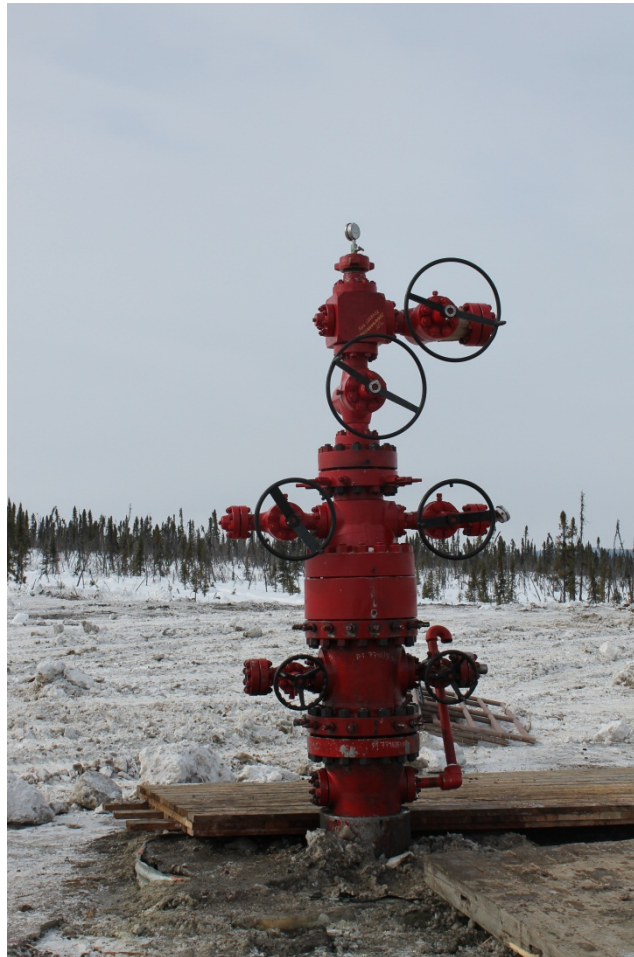
Figure 2: H-28 Wellhead Final Installation - April 16 th 2013
