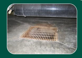
Sumps and Rock Pits - water carrying hydrocarbons and solvents that enter the sump may contaminate the groundwater
