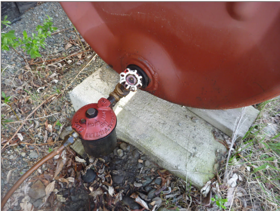
Photo 6: Hydrocarbon staining around AST located at the Youth Drop-In Center
