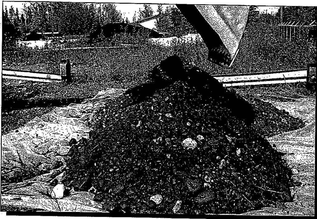
Photo 2 Stockpiled soil from UST excavation
